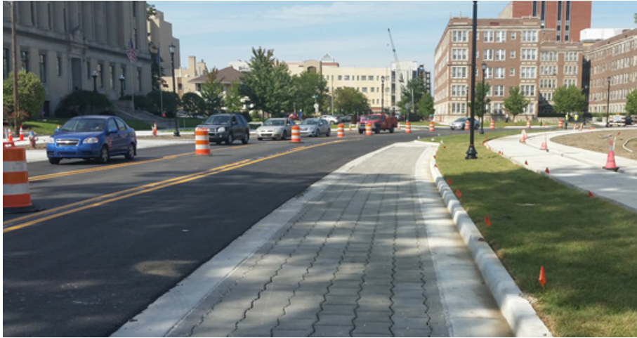
4' Permeable Pavement on Each Side of Street Stone Reservoir Across Full Roadway
