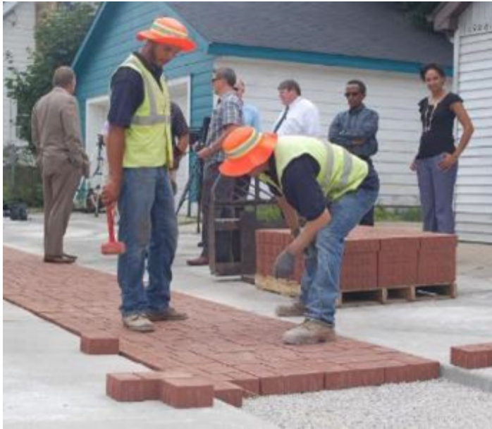
3 ft Wide Center Strip of Permeable Pavers, Full Length of Alley
