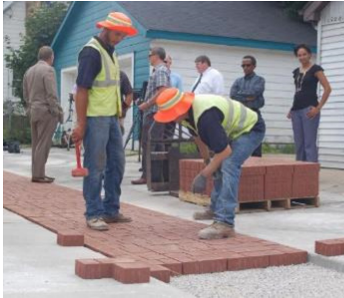
3 ft Wide Center Strip of Permeable Pavers, Full Length of Alley or Catch Basins (not shown)
